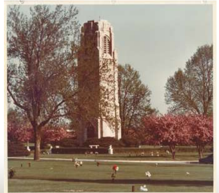
Tower with surrounding concrete fixtures and hedges.
