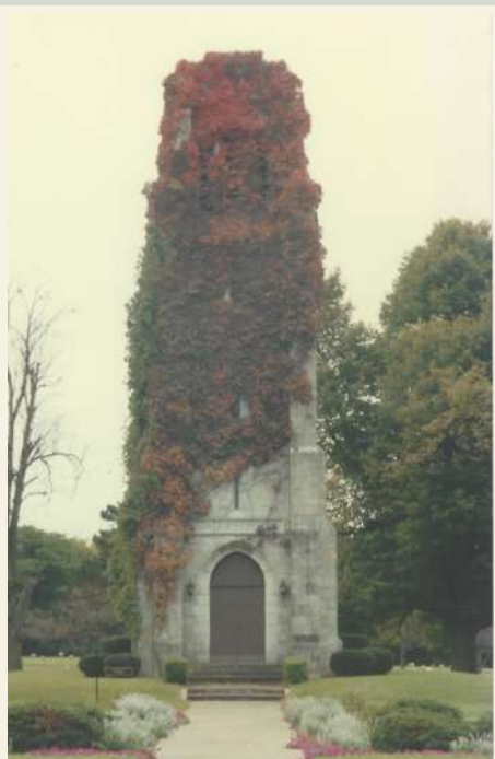
Tower in 2000 with ivy vines
